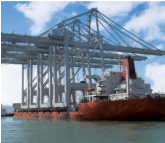
Photo: Super Post-Panamax Ship-to-Shore (STS) Cranes being delivered to Barbours Cut Container Terminal, May 2015. New STS cranes are an important part of the \$700 million modernization project underway at Barbours Cut to accommodate the significantly larger vessels calling the terminal. On the waterside; the terminal channel has been deepened to 45 feet to match the depth of the federal Houston Ship Channel.
