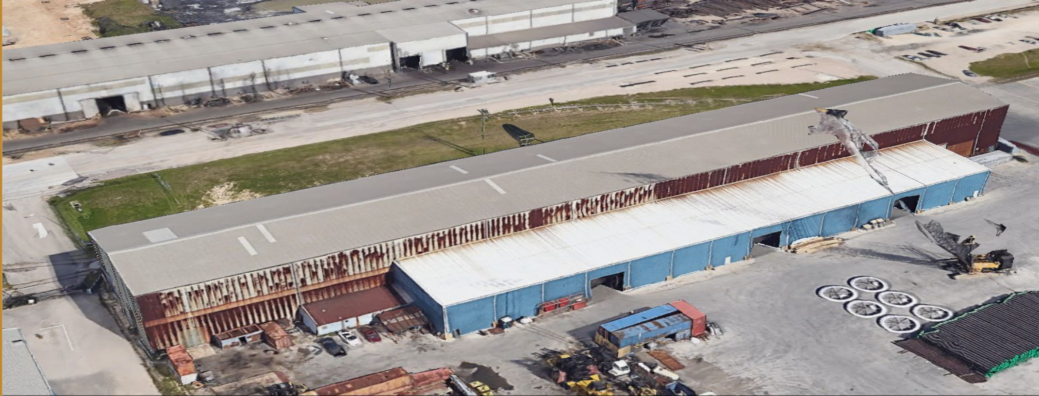
Installation of new overlay roofing system on top of existing roof.
