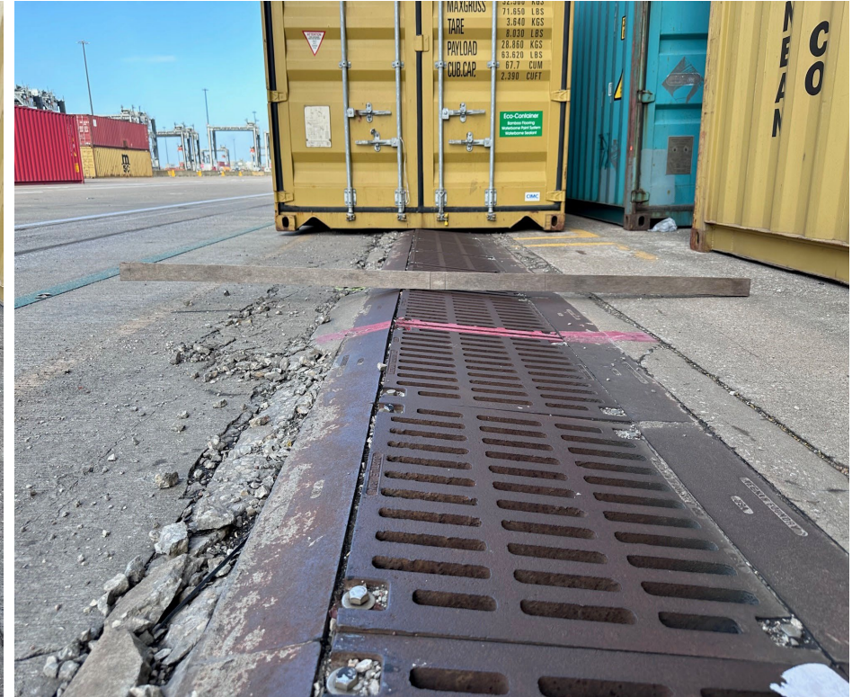
Repair of existing trench drain, including demolition, concrete repairs, concrete pavement replacement and new pavement markings.
