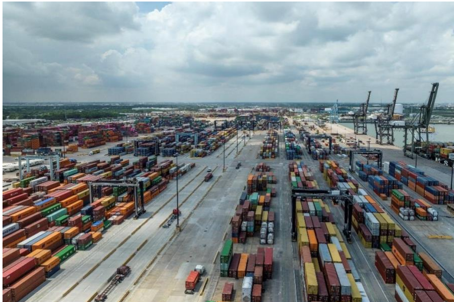
Barbours Cut Container Terminal, Port Houston
