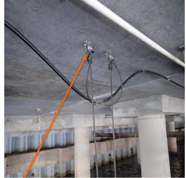
Typical Anode support in good condition
