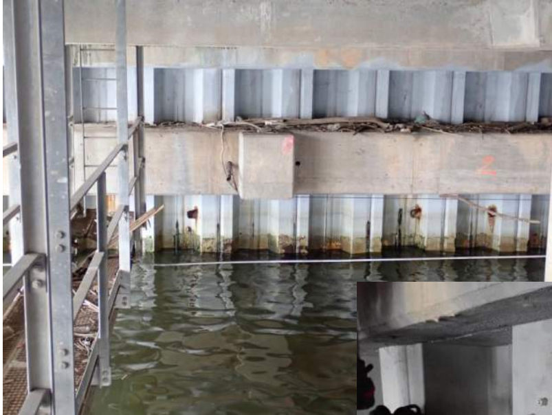
Epoxy Coating at Bulkhead Wall
