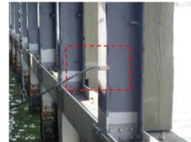
Figure 7. Connection bond from the bulk head wall to the fender piles, no major visible signs of corrosion or distress.
