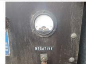
Figure 1. Broken ammeter displaying 0 amps of current
