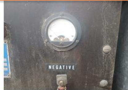
Figure 1. Broken ammeter displaying 0 amps of current
