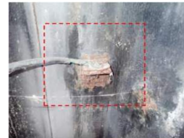
Figure 8. Negative wire connection from rectifier to bulkhead wall, showing visible signs of corrosion at connection point.
