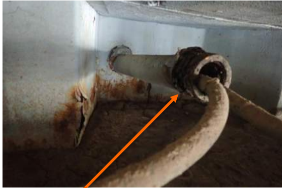
Typical condition of CS conduit, protecting wiring
