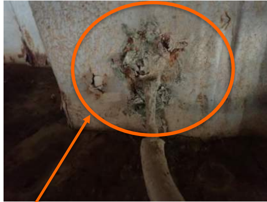
Negative structure connection exhibiting moderate corrosion
