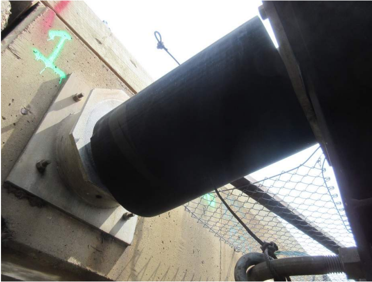
Figure 4. Displaced damper at Bent 1.
