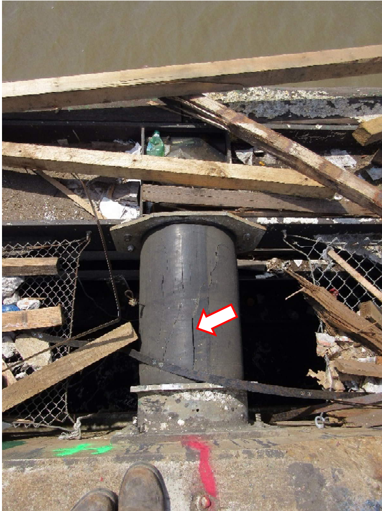
Figure 5. Severely cracked damper at Bent 4 (arrow).
