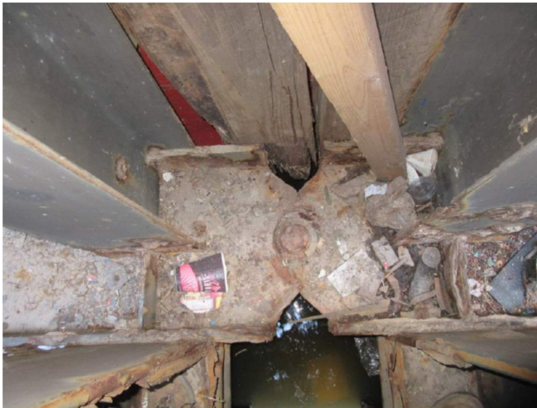
Figure 14. Bent 11 secondary framing pinned connection
