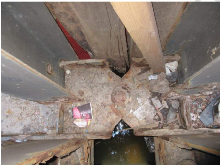
Figure 14. Bent 11 secondary framing pinned connection
