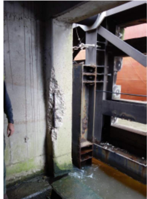
4' x 2' Spall due to corrosion; photo # 747-014
