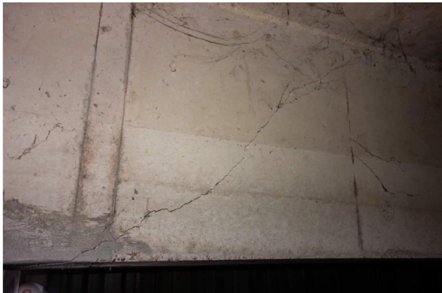
Figure 7. Deck beam shear crack
