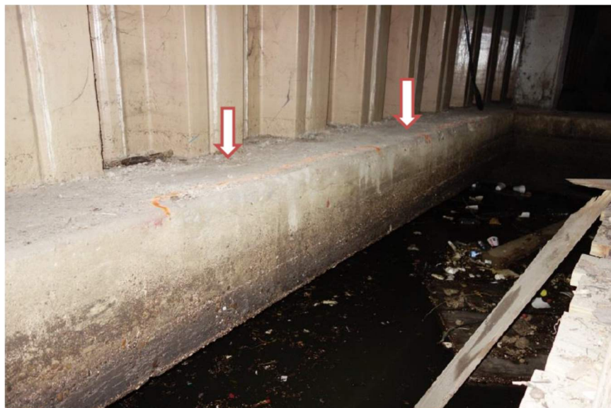
Figure 13. Delamination on tieback whaler
