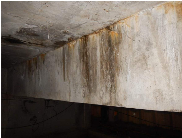
Figure 6. Crack at beam to deck transition
