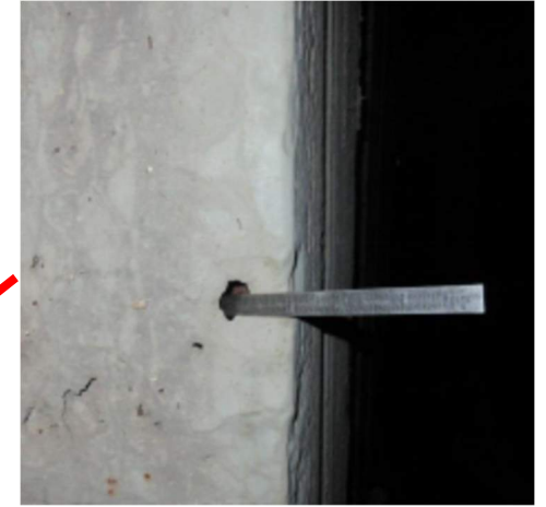
1 SF steel bulkhead wall corrosion; photo# 747-013
