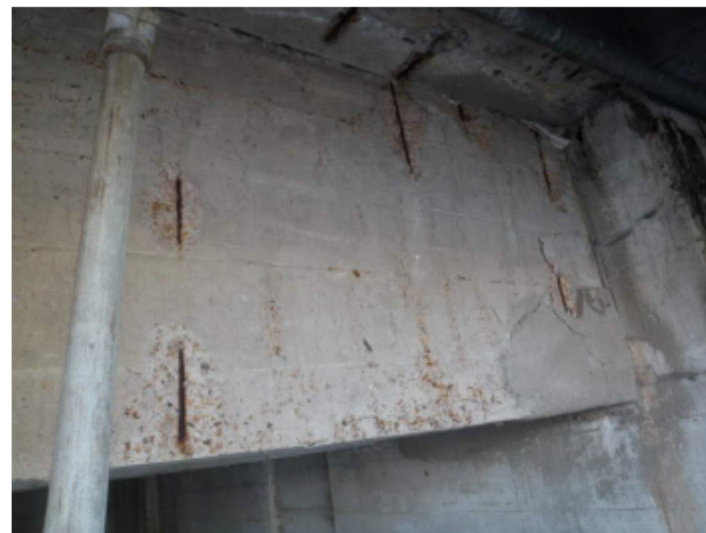
36" x 8" spall due to corrosion; no observed reinforcing steel section loss photo # 747-009
