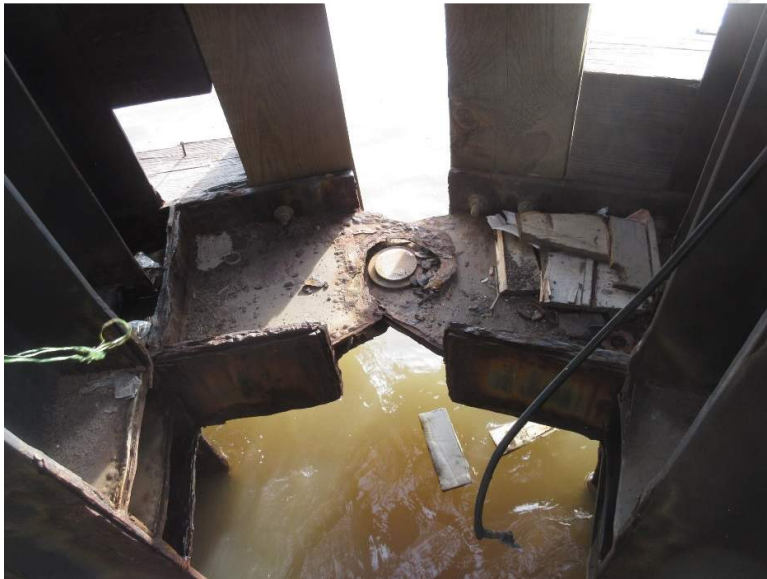
Figure 7. Failed pin connection at joint in secondary framing at Bent 26.
