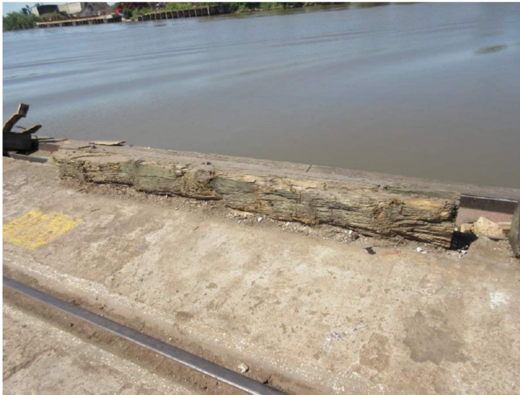
Figure 15. Typical wharf log distress
