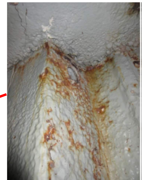
3' long x 2' tall area steel bulkhead wall corrosion; photo # 747-012
