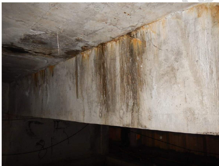
Figure 6. Crack at beam to deck transition
