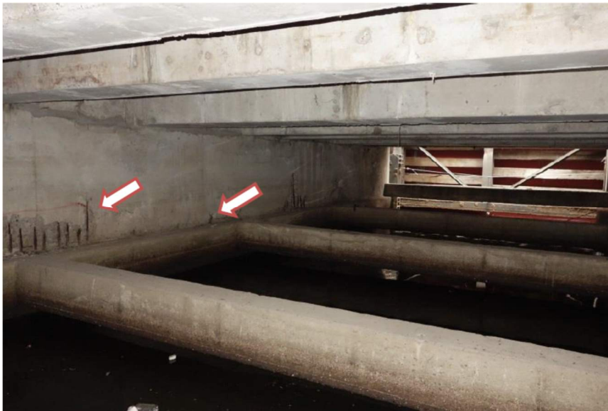
Figure 10. Spalling at RC Shear Wall
