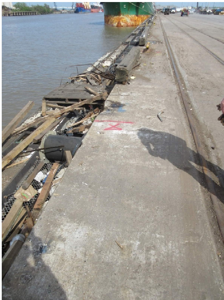
Figure 10. Missing wharf log near Bent 4.
