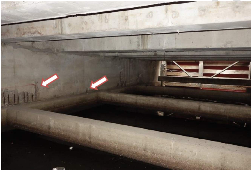
Figure 10. Spalling at RC Shear Wall
