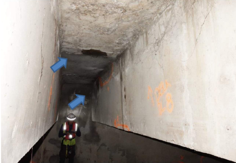
Figure 5. Beam bottom spall and delamination
