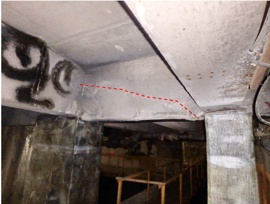
Figure 1. Elevation of damaged shear wall section above opening (red dashed line).
