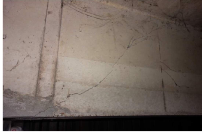
6 LF crack causing no reduction in capacity; photo # 747-011
