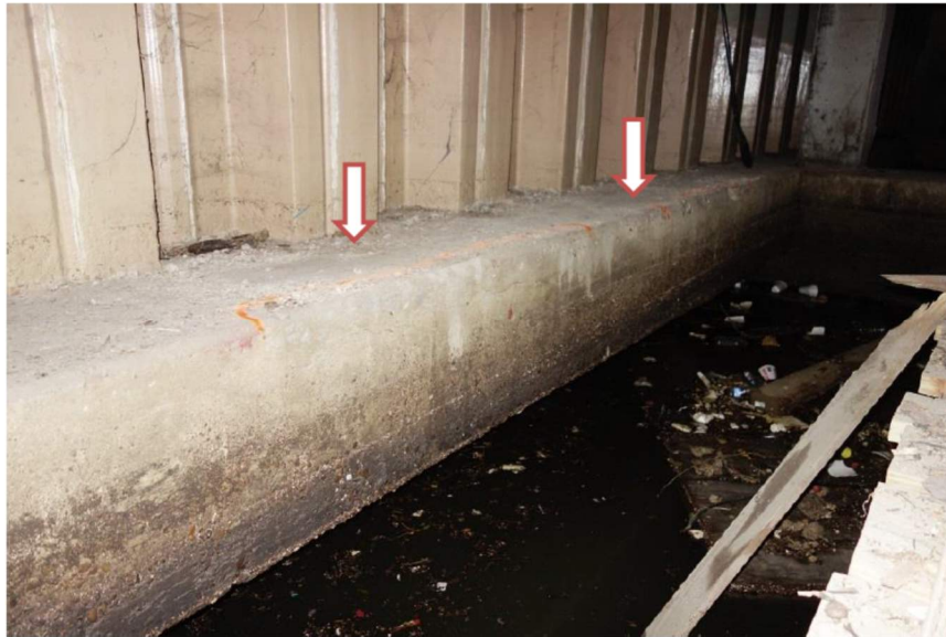
Figure 13. Delamination on tieback whaler
