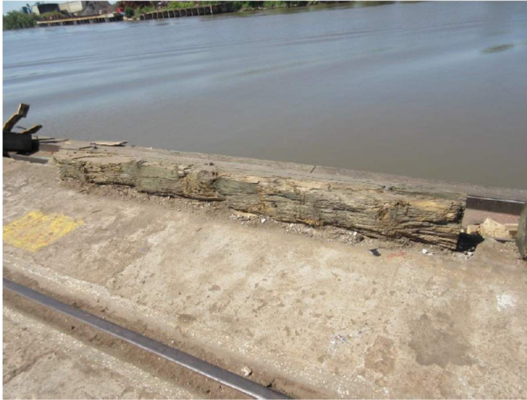
Figure 15. Typical wharf log distress
