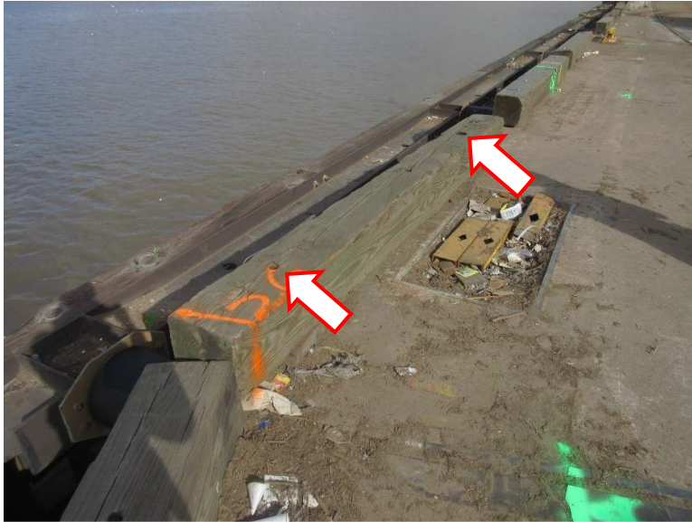
Figure 11. Wharf log with missing anchors near Bent 26 (arrows).
