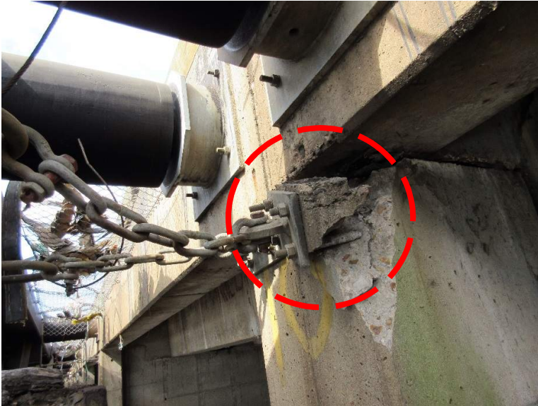
Figure 8. Failed stay chain anchorage at Bent 10 (red dashed circle).
