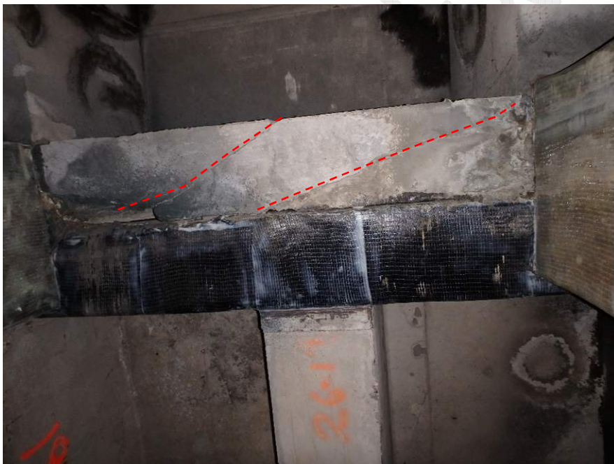
Figure 2. Soffit of opening through shear wall exhibiting shear cracks (red dashed line).
