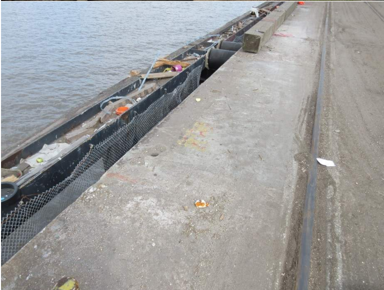
Figure 9. Missing wharf log near Bent 18.
