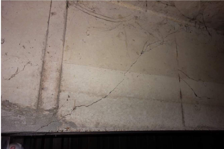
Figure 7. Deck beam shear crack
