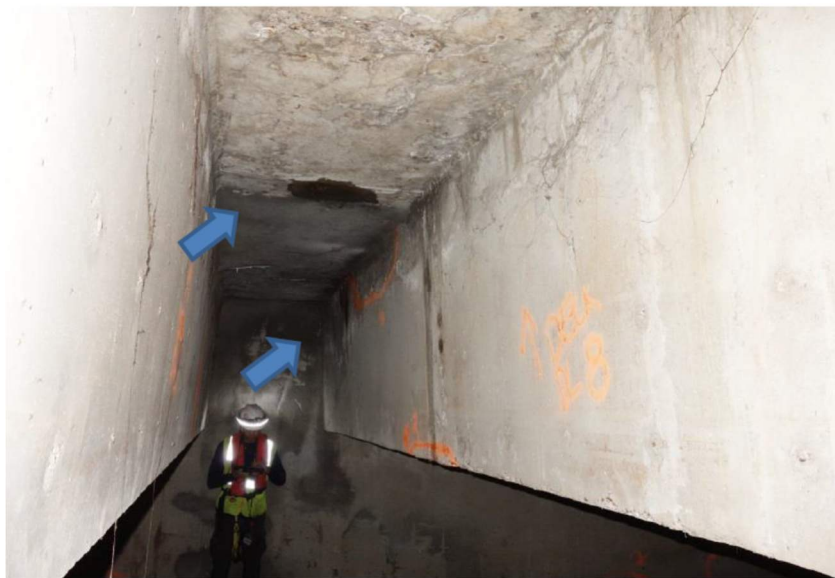
Figure 5. Beam bottom spall and delamination
