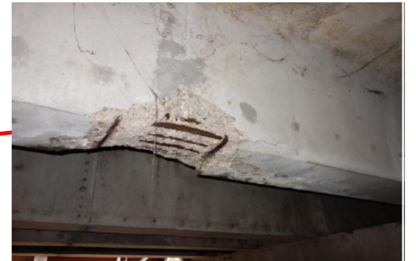
2 LF Spall due to corrosion; measurable reinforcing steel section loss with w/further review required due to rebar section loss; photo # 747-006
