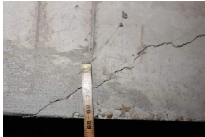
4 LF causing reduction in flexural capacity; photo # 747-010
