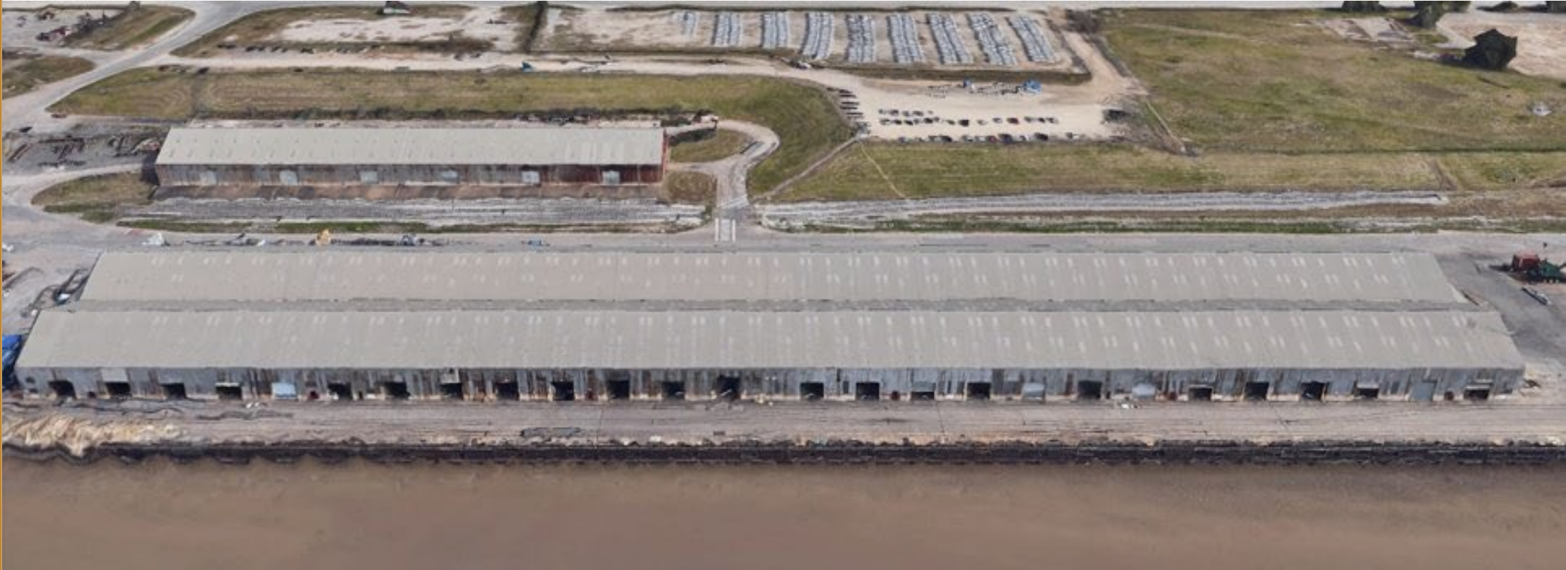
Overlay of new roofing system over existing roof.
