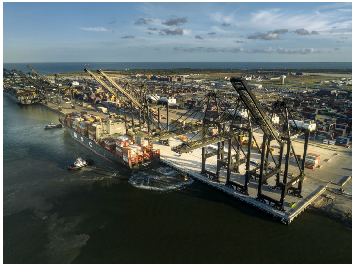
Wharf 6 at the Bayport Container Terminal is now fully operating, adding much-needed cargo volume capacity at the two fastest-growing container terminals in the Gulf.
