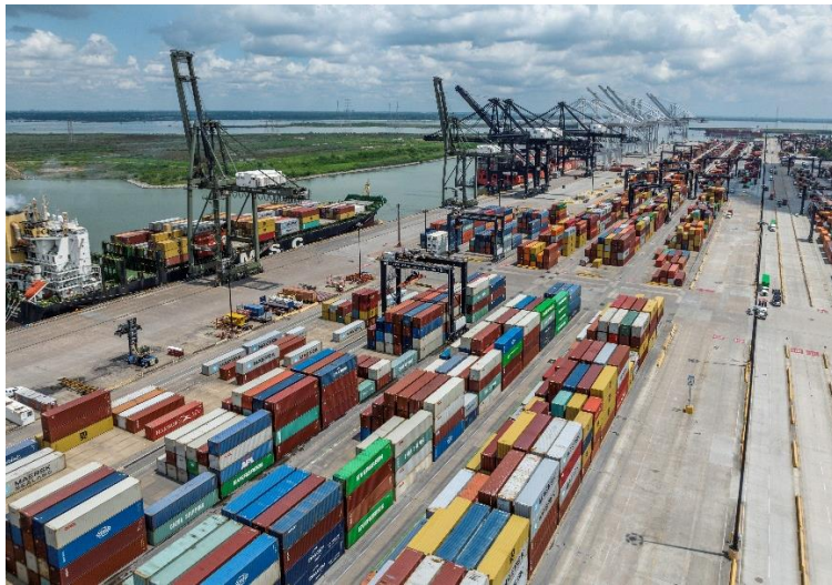
Port Houston's Barbours Cut Container Terminal
