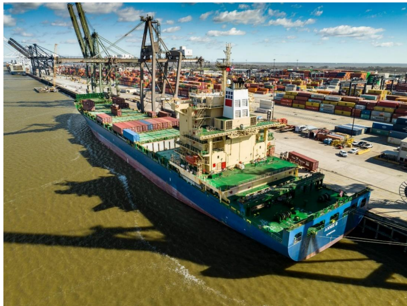
Port Houston's Barbours Cut Container Terminal
