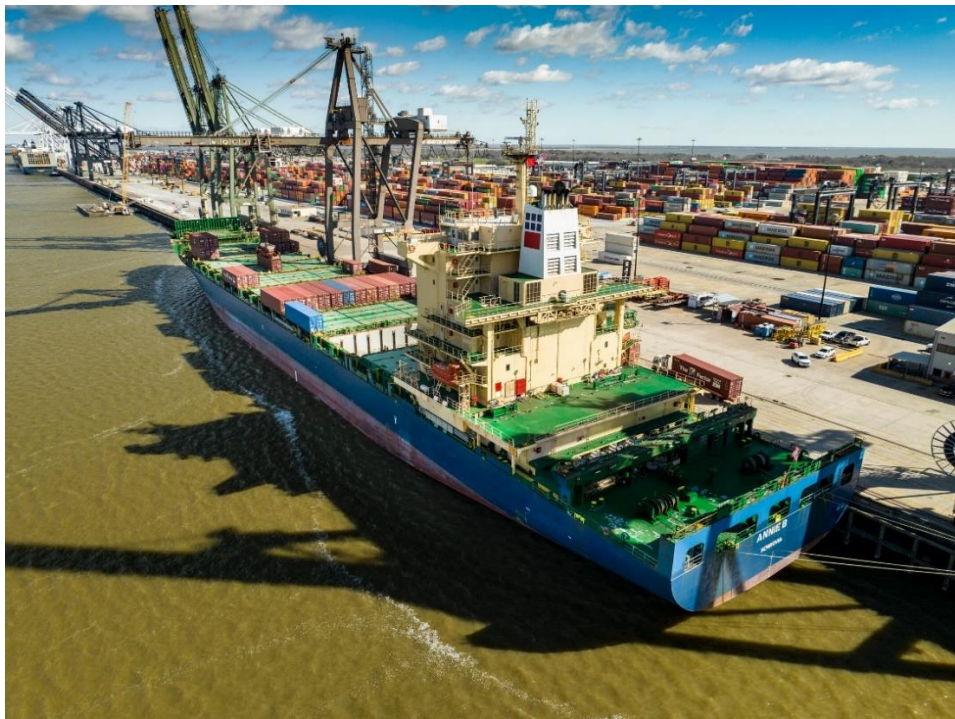
Port Houston's Barbours Cut Container Terminal
