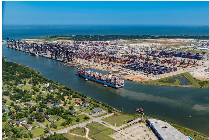
Port Houston's Bayport Container Terminal
