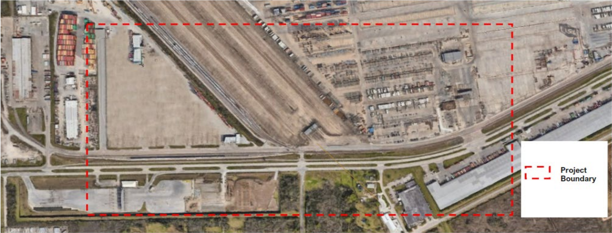
Expansion of the existing communication and power lines at the west end of Barbours Cut Terminal including additional conduit installation, boring to cross existing roads and rail tracks and pulling wire from existing termination points within the terminal.
