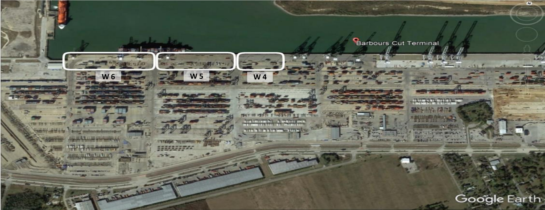
Construction of 1,333 feet of new wharf structure at the Barbours Cut Container Terminal. The project scope includes surveying, dredging, drilled shaft foundations, structural concrete, crane rails, fender systems, utilities, and a stevedore support building.
