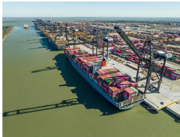
Dock side view of Bayport Container Terminal
